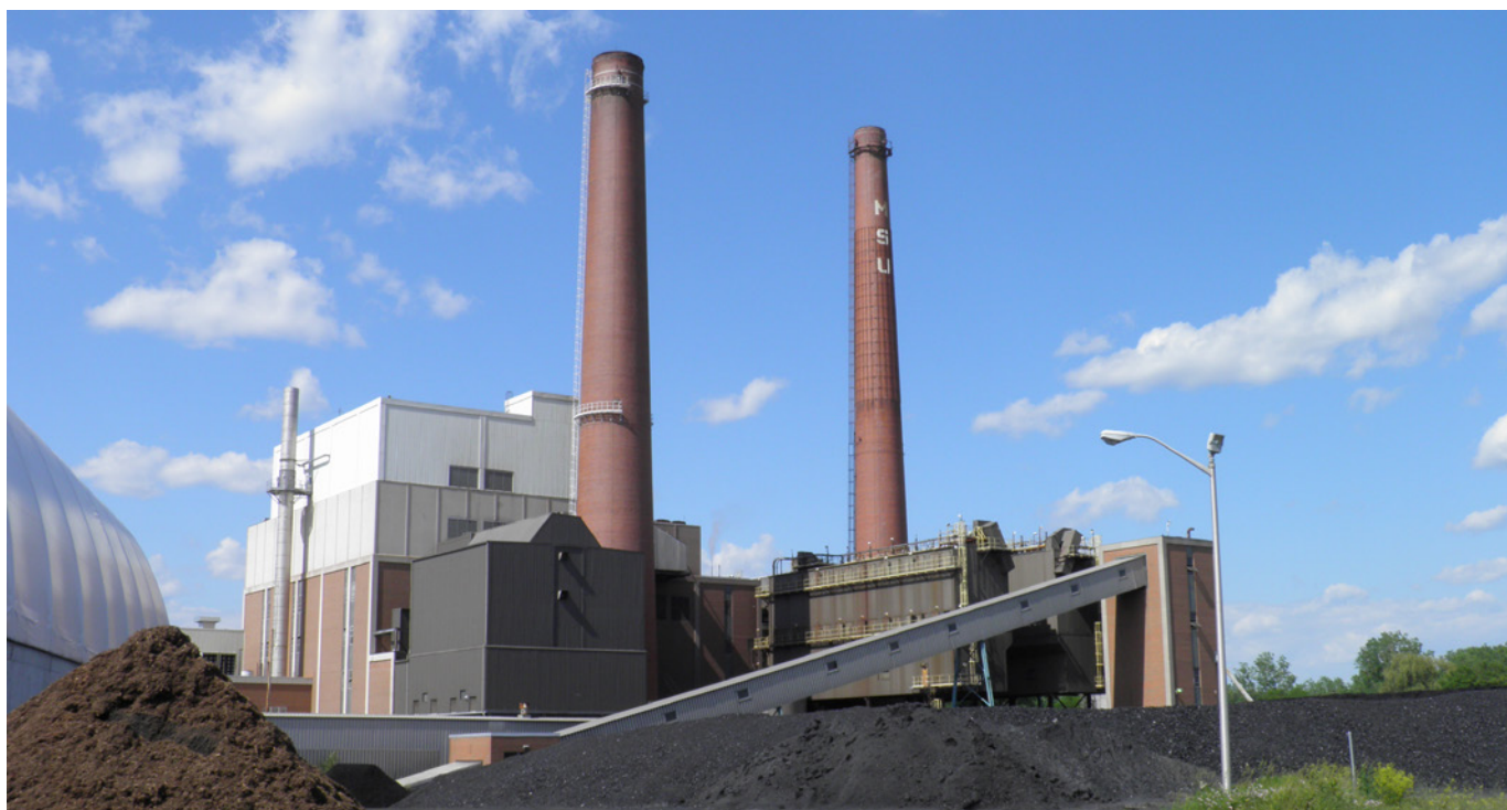
T. B. Simon Power Plant at Michigan State University. The plant provides electricity, heating, cooling, and water to the East Lansing campus. Its primary fuel is coal. Photo © Michael P. Kube-McDowell
