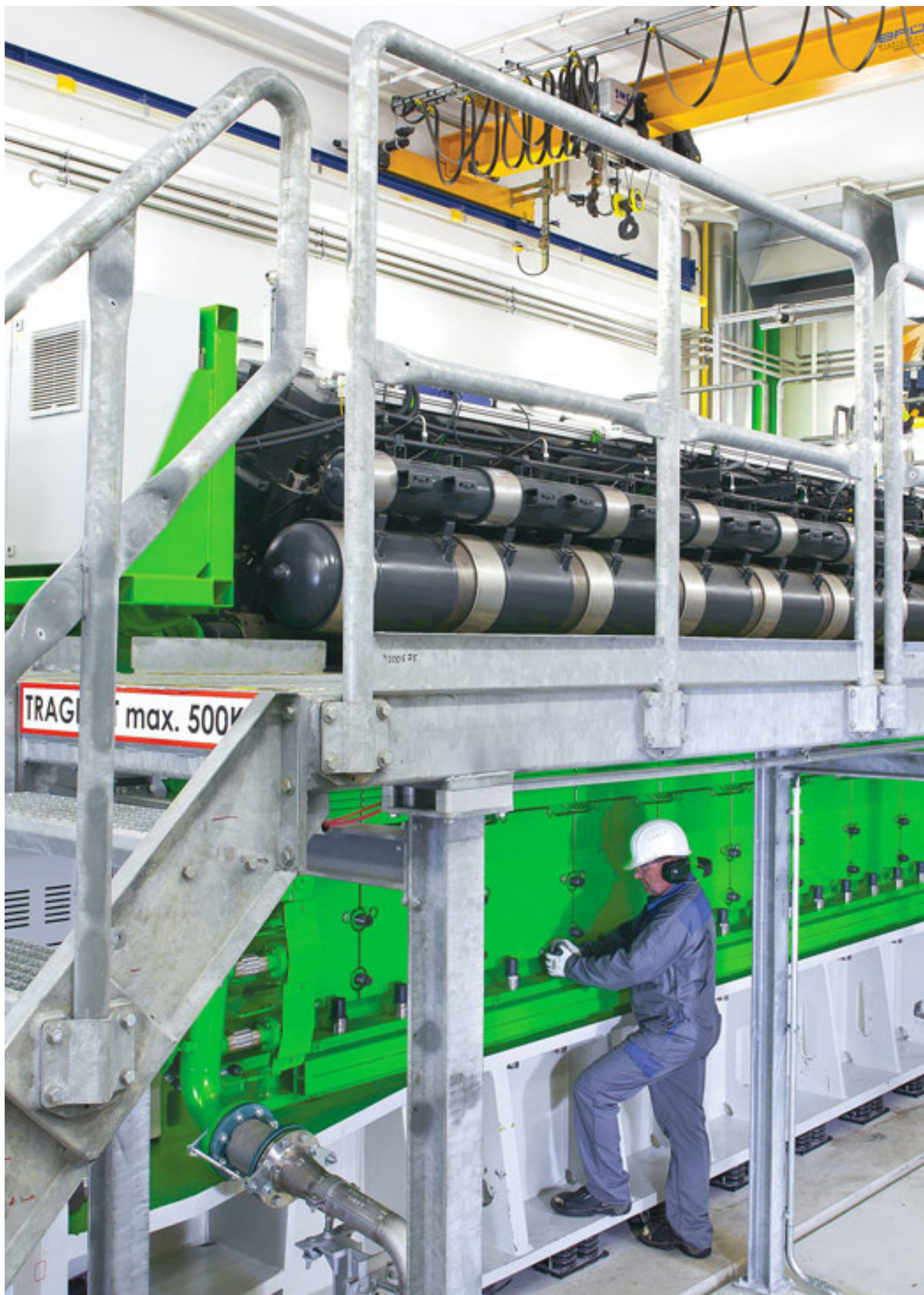
The municipal utility in Rosenheim, Germany counts on a Jenbacher J920 FleXtra cogeneration plant to provide high efficiency heat and power to the citizens.
