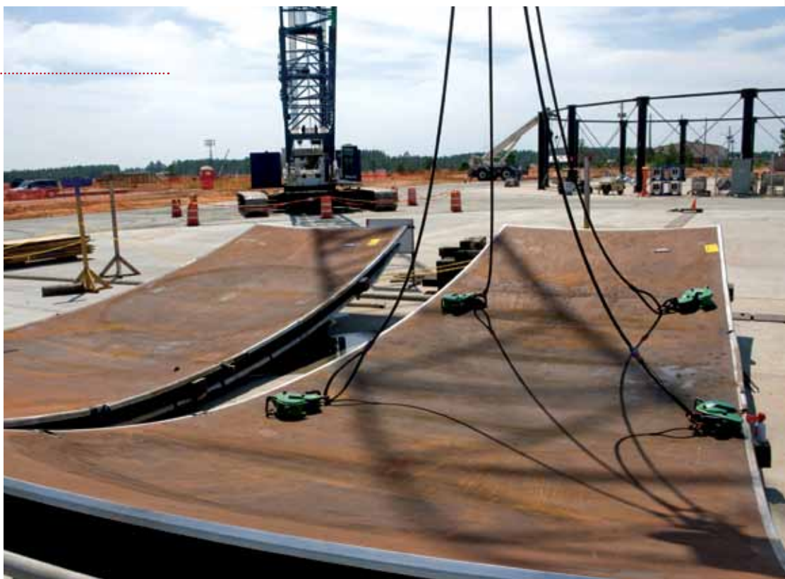
First containment vessel plates arrive for Plant Vogtle Units 3 and 4, September 8, 2010.
