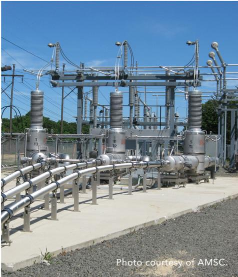
Long Island Power Authority (LIPA) is utilizing a cable system manufactured by Nexans that utilizes AMSC's HTS wire and an Air Liquide cooling system. Energized in April of 2008, this is the world's first superconductor transmission-voltage cable system and is capable of transmitting up to 574 megawatts (MW) of electricity and powering 300,000 homes.
