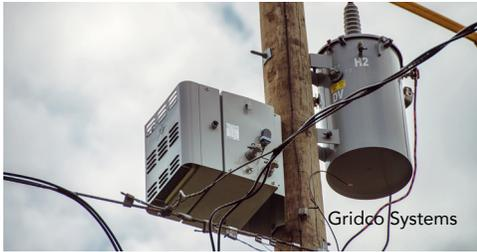
Voltage and Volt-Ampere Reactive (VAR) Optimization (VVO) is a smart grid-enabled utility application. VVO controls the flow of power on the distribution system to increase efficiency and reliability, reduce distribution energy losses, and accommodate new power flows, such as those originating from distributed generation. By providing more precise voltage control, VVO reduces total energy consumption without compromising service quality.
