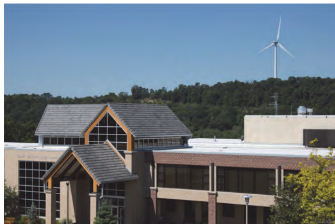
Figure 7-2. Luther College's wind turbine on campus.
