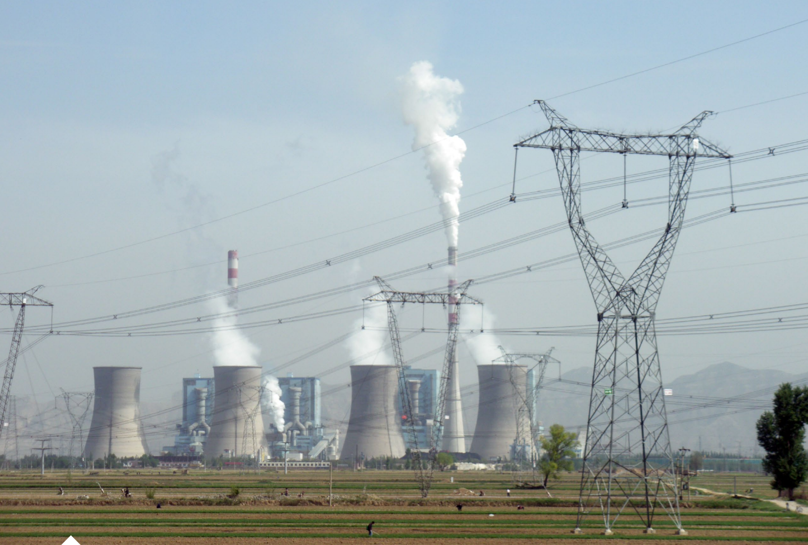
Photo of a coal-fired power plant in Shuozhou, Shanxi, China. Photo credit: Kleineolive/Wikimedia.
