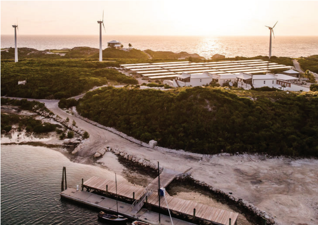
Installation: Over Yonder Cay — (The Exumas, Bahamas)
