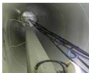
Cabling and grid connection
