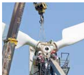
Dismantling the project
