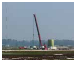
Site preparation and civil works
