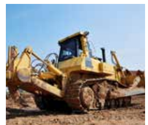
Clearing the site
