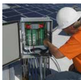
Cabling and grid connection
