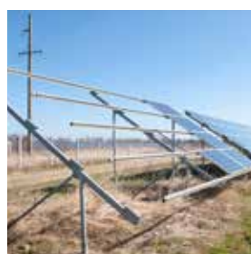
Dismantling the project
