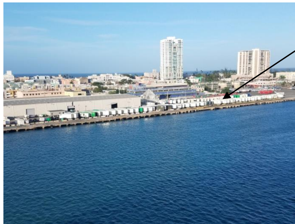
Diesel generators Fuel Trucks
