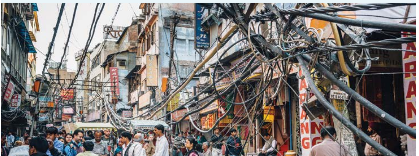
Photo of electric cables on the streets of Old Delhi.
