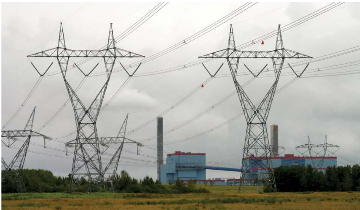
Photo courtesy David Dodge, The Pembina Institute. Genesee coal-fired power plant in Alberta.
