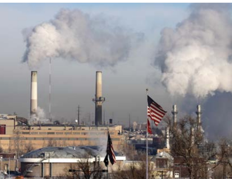
Arapahoe Station Coal fired power plant Denver Colorado
