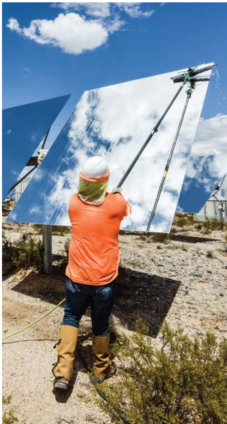
Photo courtesy Dennis Schreeder for NREL. Contracted workers clean Heliostats at the Ivanpah Solar Project.
