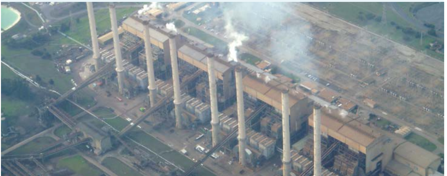
Photo courtesy Mriya for WikiCommons. Hazelwood Power Station as seen from a light aircraft flying overhead.
