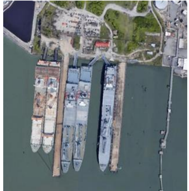
Figure 24 Aerial image of 1201 Terminal Avenue.
