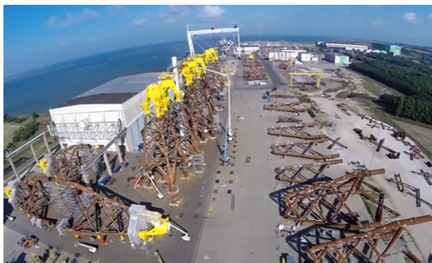
Figure 10 Bladt Industries jacket manufacturing, Denmark.
