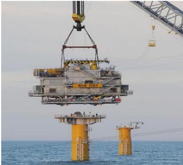
Figure 11 Offshore substation being installed at Sheringham shoal OSW farm (UK).
