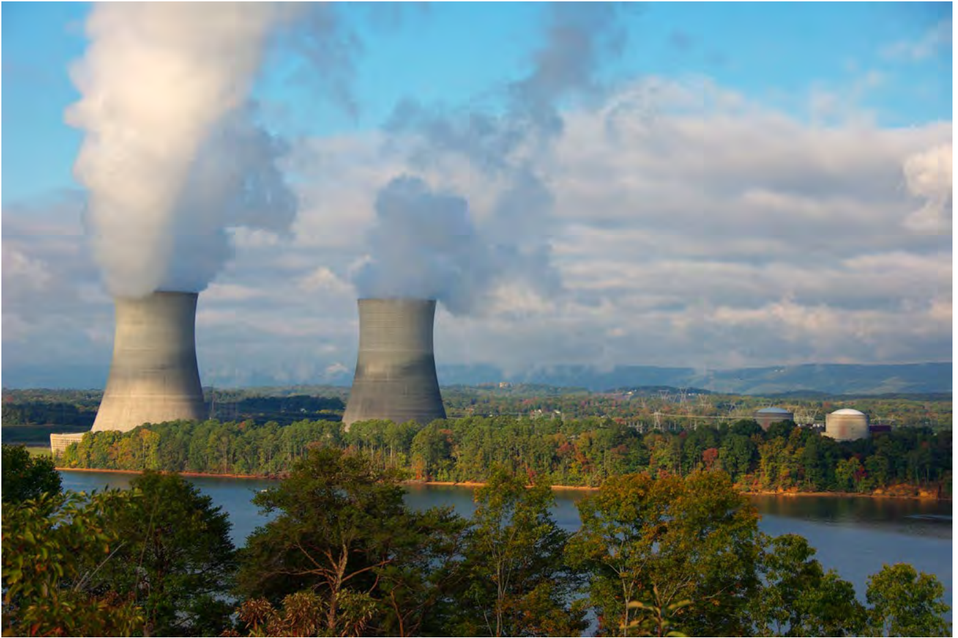
Sequoyah Nuclear Power Plant near Chattanooga, Tennessee, October 25, 2008. Source: Wikimedia Commons/ Photorush.
