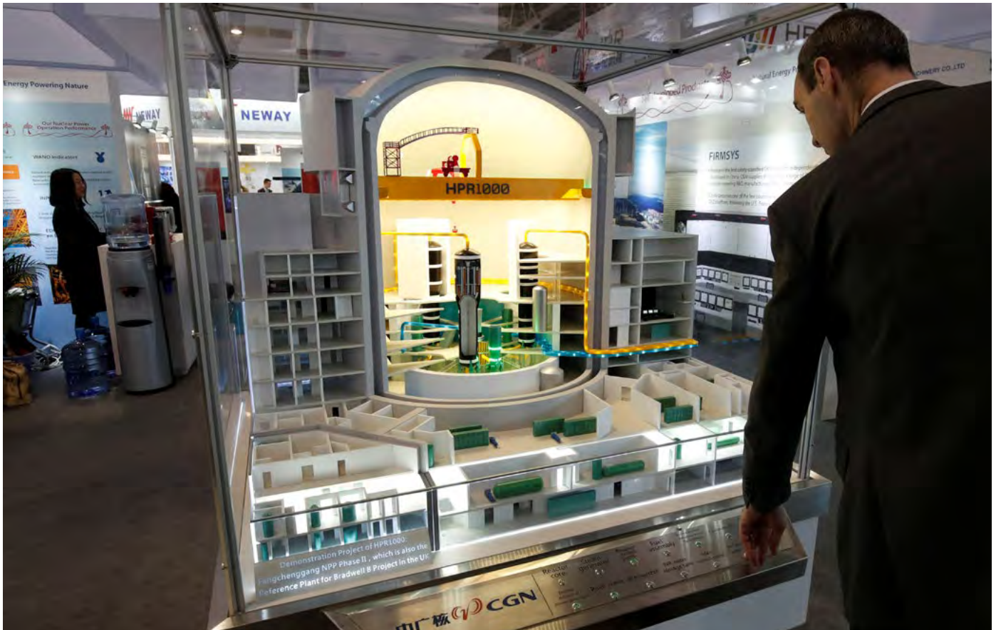
A cut-away model of the Chinese Gen-III nuclear power technology Hualong 1 by China General Nuclear Power Corporation (CGN) is displayed at the World Nuclear Exhibition (WNE), the trade fair event for the global nuclear community in Villepinte near Paris, France, June 26, 2018. Source: REUTERS/Benoit Tessier.
