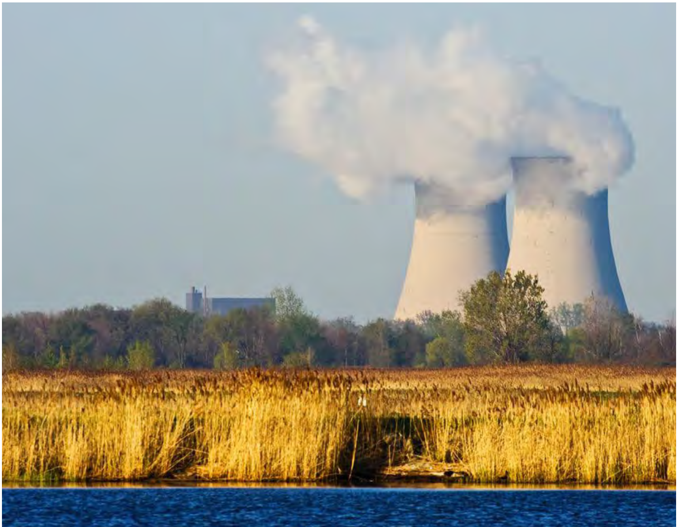
Enrico Fermi Nuclear Power plant on Lake Erie, Rockwood, Michigan. May 2008. Source: James Marvin Phelps/Flickr.
