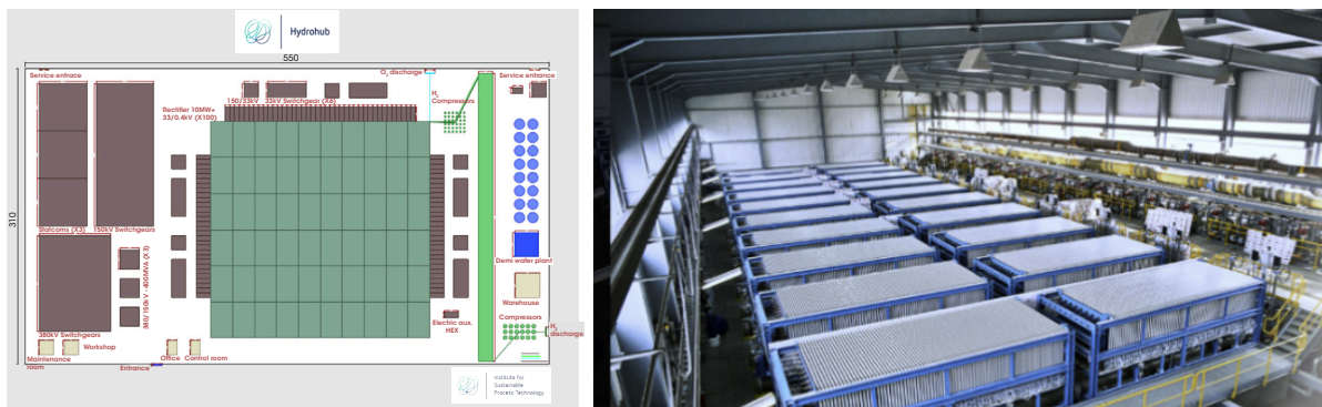
Figure 13. Plot size for an alkaline 1-GW electrolyser plant (left) and for a 100-MW alkaline electrolyser from Thyssenkrupp (right).
